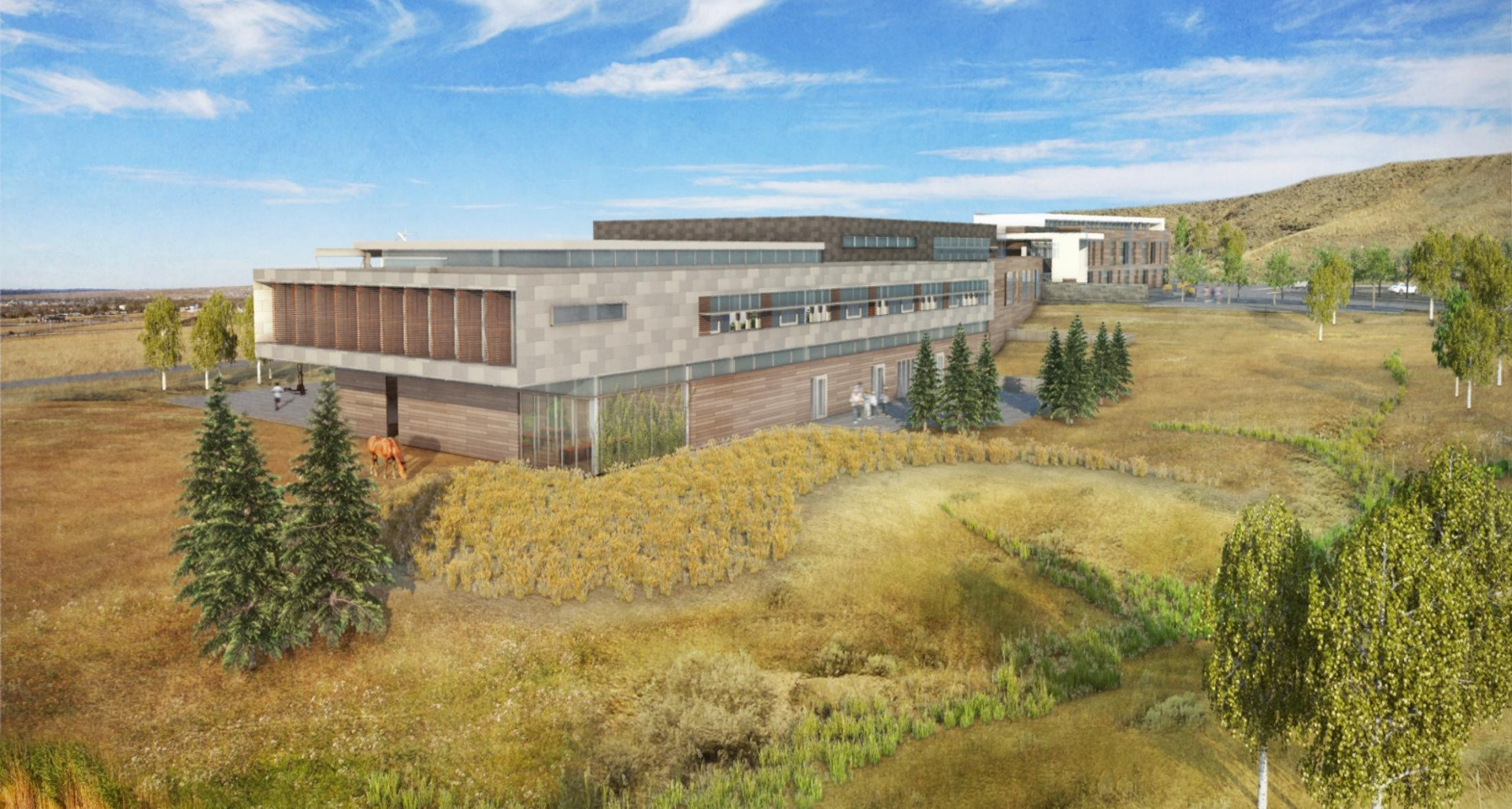
New High School Campus: Center for Advanced Professional Studies & Roosevelt HS Natrona County School District, Casper WY
