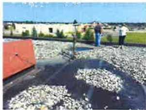
North side main roof
