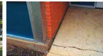
Brick ledge and glazing
