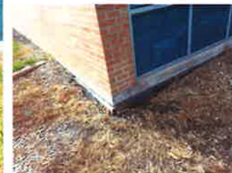
Exposed base of wall
