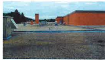
North side main roof
