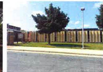
Original north wing
