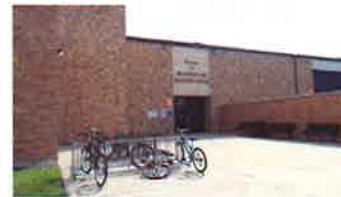
West Entry- primary student entry
