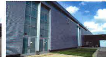
Gym metal cladding with glazing above doors
