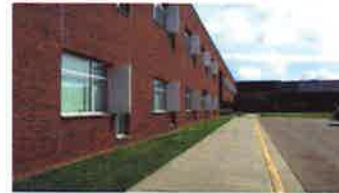
Brick exterior - west exposure
