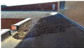
North side main roof
