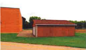
Storage building exterior
