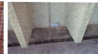
Original north wing
