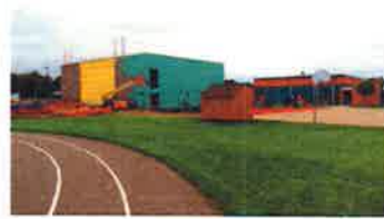
Addition under construction
