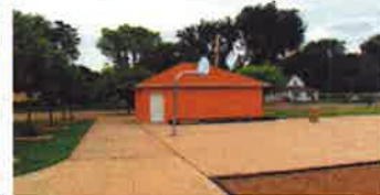
Storage building exterior
