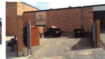
Loading Dock and trash enclosure
