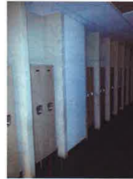
Hallway with lockers -1993 addition
