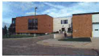
West addition and loading
