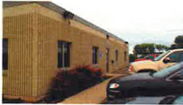
West, Main Entry
