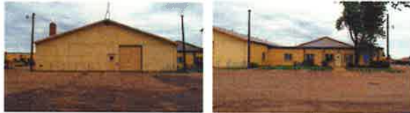
South face, west side
