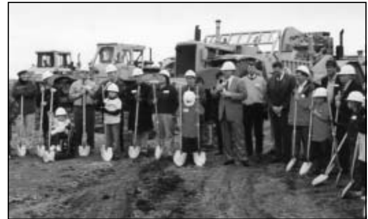
Dr. Larry P. Nybladh, superintendent, reminds the crowd gathered for the groundbreaking that it is the responsibility of each generation to provide for the next.
