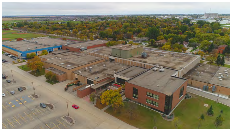
Northwest aerial view of High School | October 2018
