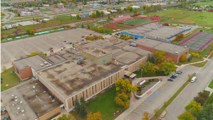
Southwest aerial view of High School | October 2018
